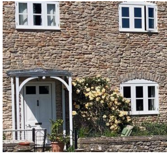
Traditional windows and door with porch
