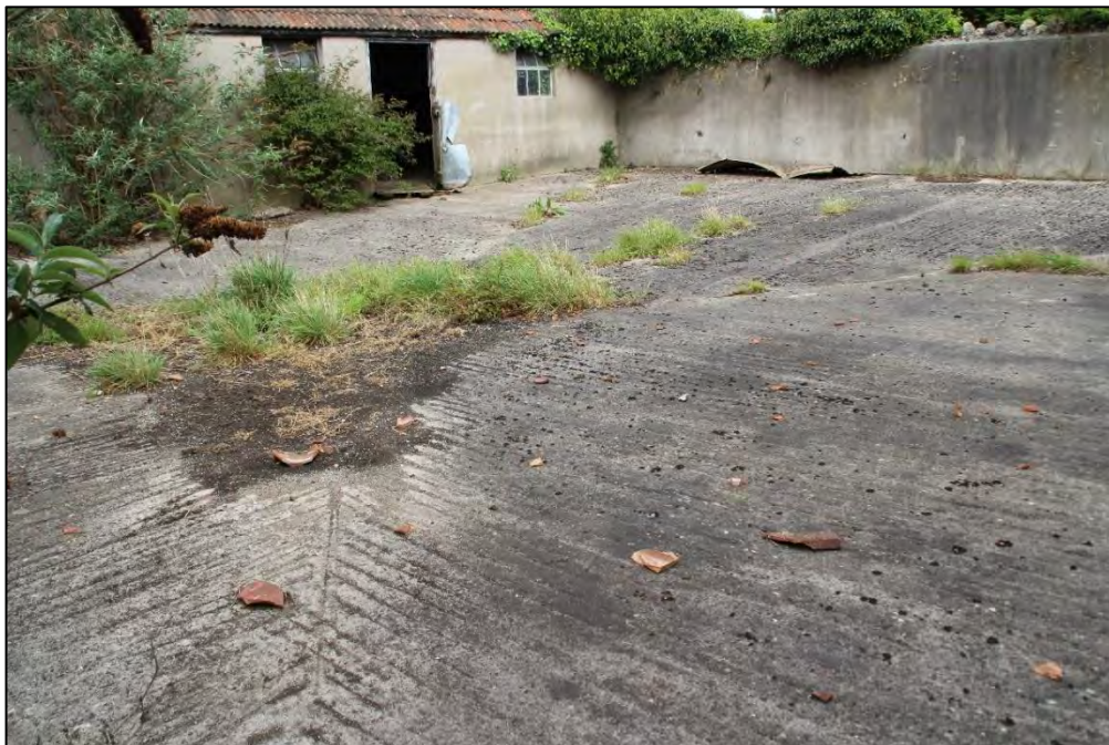
Photo 34 The courtyard cement ground surface
