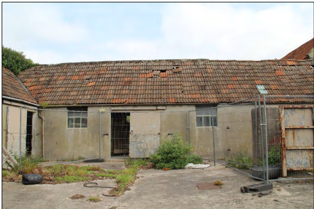
Photo 12 The southern elevation of Building A, western section
