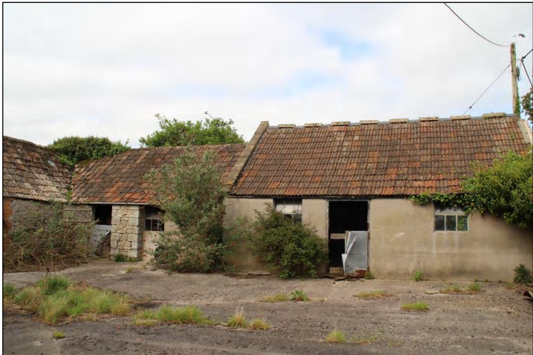
Photo 15 Building B seen from the east looking west
