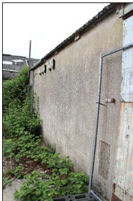
Photo 27 Detail of the eastern wall of Building D
