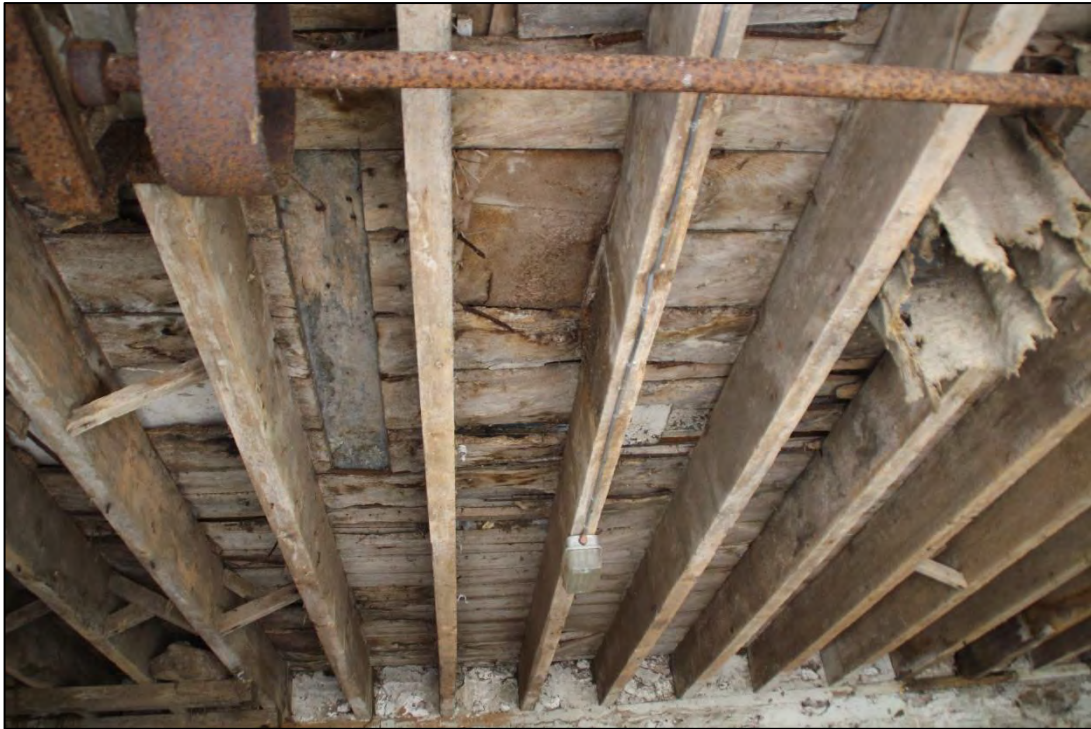
Photo 9 Detail of the first-floor structure
