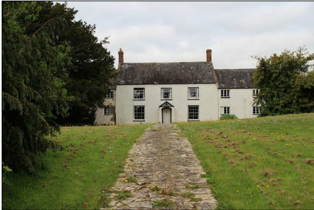
Photo 35 Grade II Listed Court House Farmhouse (A), viewed from the east
