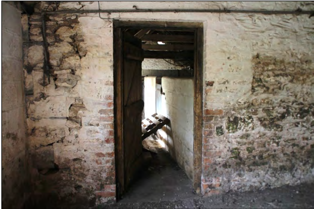
Photo 20 View looking into Building C from Building B
