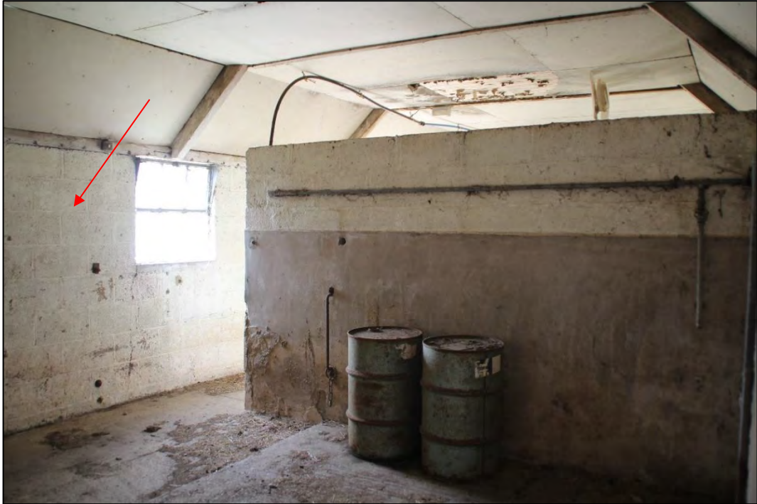
Photo 13 The interior of Building A, with concrete block southern wall arrowed
