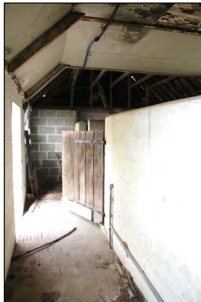
Photo 14 Interior of Building A looking west
