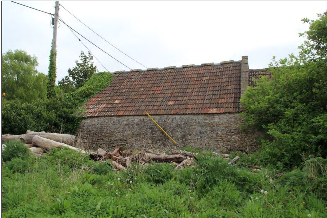
Photo 16 Building B seen from the west looking east
