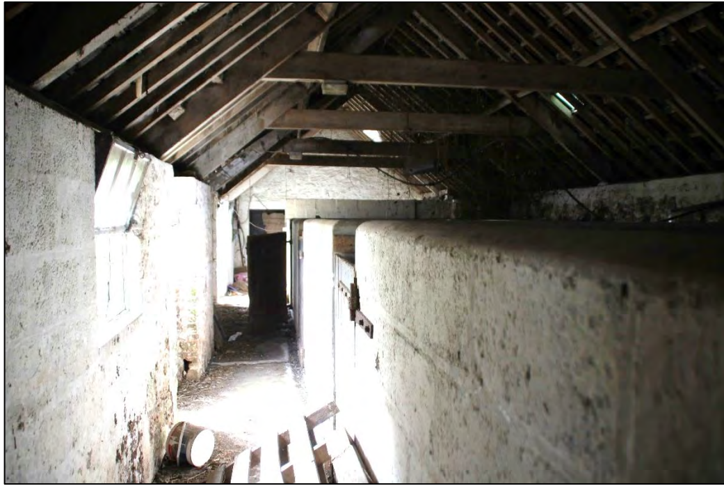
Photo 24 Internal view of Building C looking south
