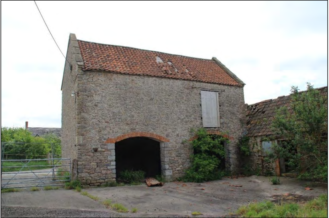
Photo 7 The granary viewed from the west looking east
