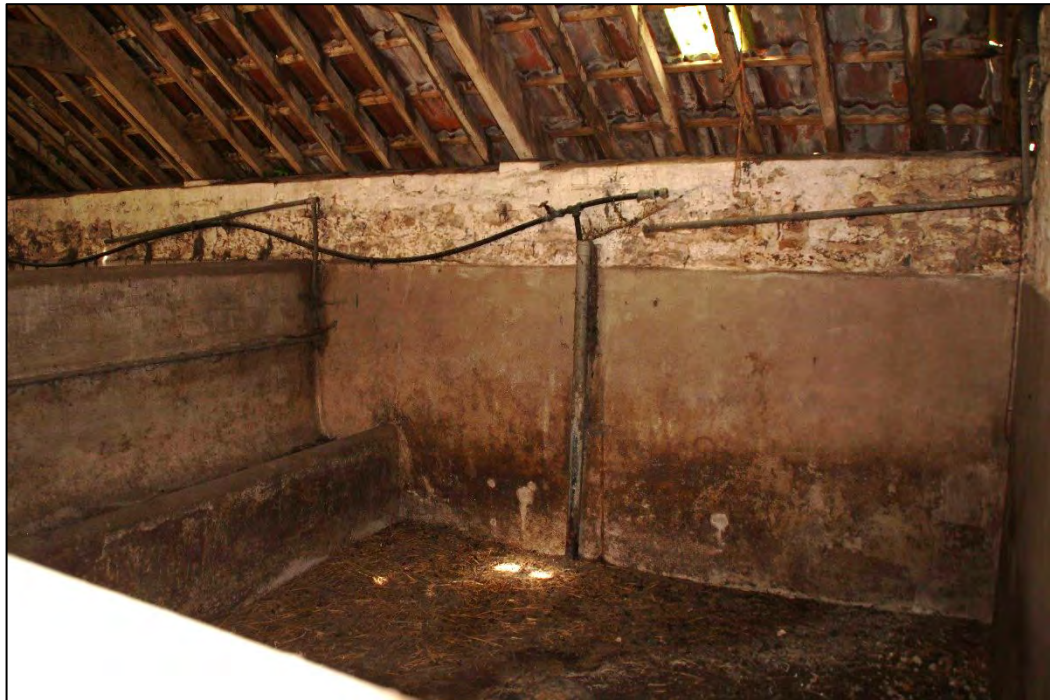
Photo 25 Internal view of stall in Building C
