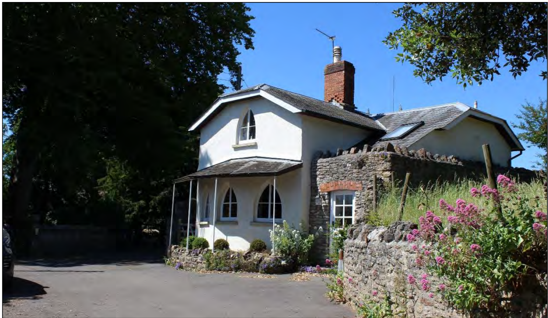
Photo 40 Grade II Listed The Lodge (D), viewed from the north-east
