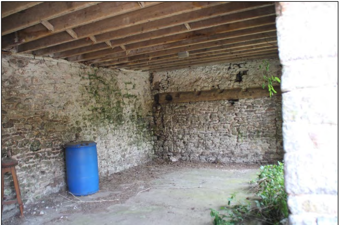
Photo 8 The interior of the granary cart shed
