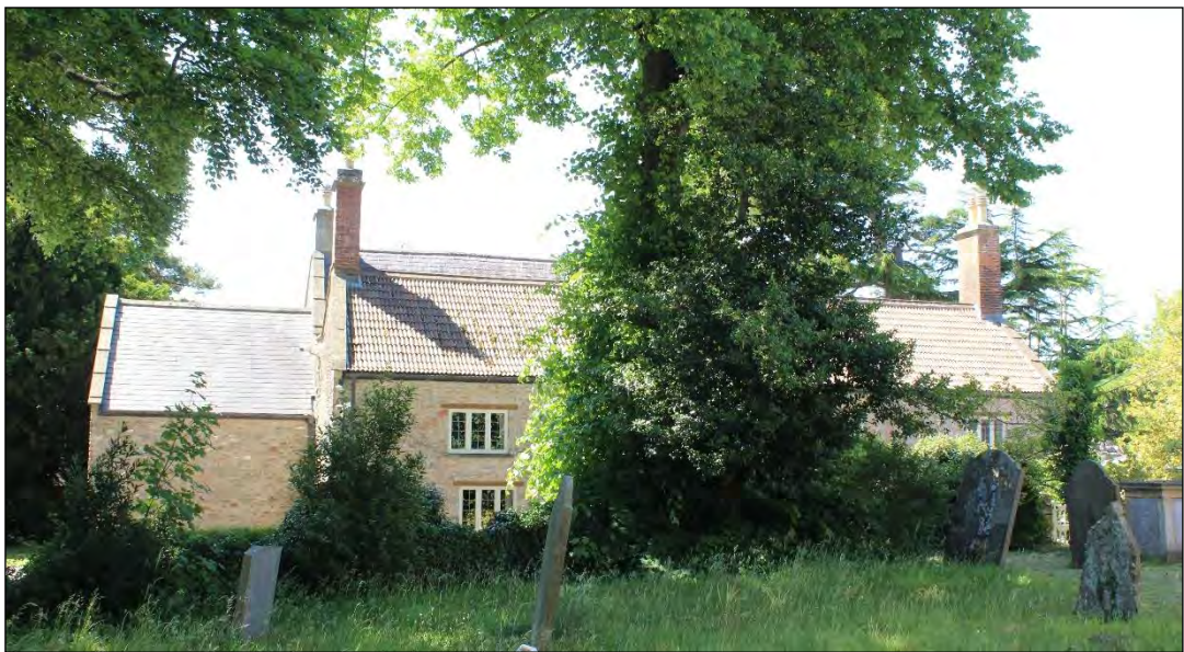
Photo 37 Rear of the Grade II Listed Westbury House, viewed from the east from within the churchyard
