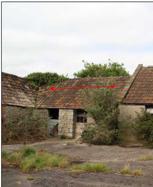
Photo 22 View of Building C from the courtyard
