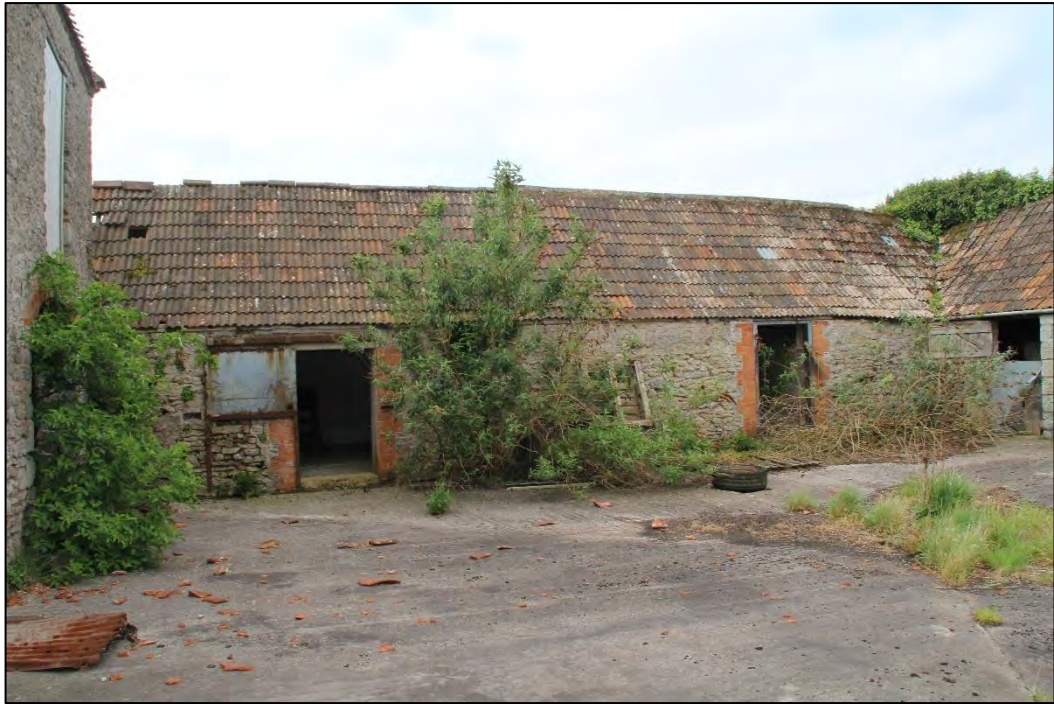
Photo 10 Building A viewed from the north looking south
