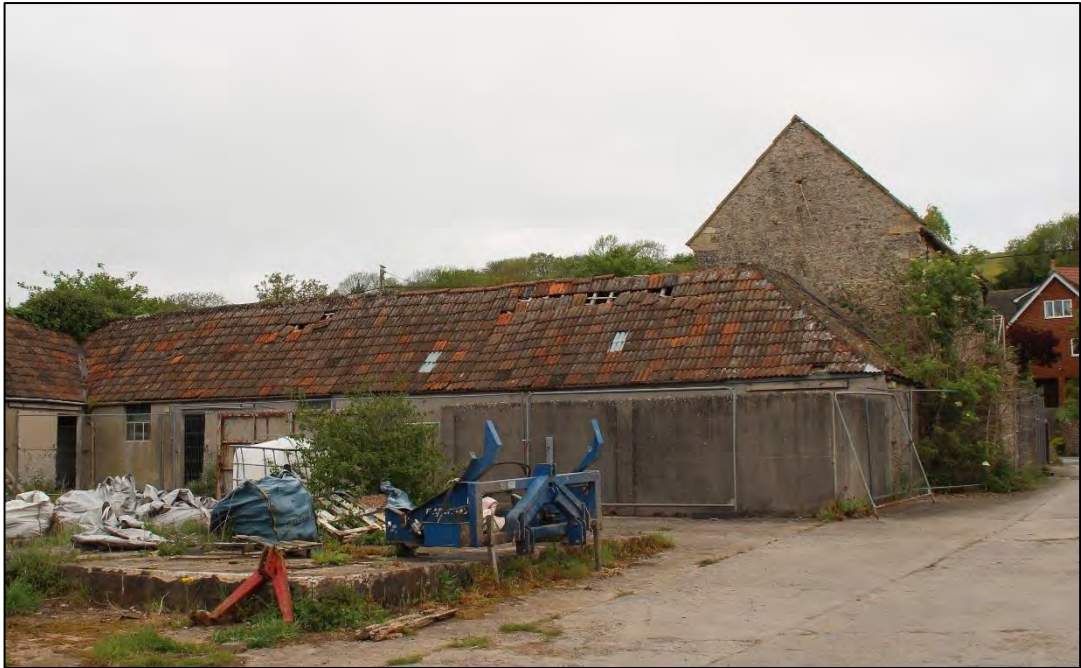
Photo 11 The southern elevation of Building A
