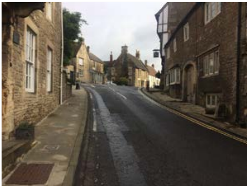
Traffic 'Pinch point' at junction of A366 and B3110
