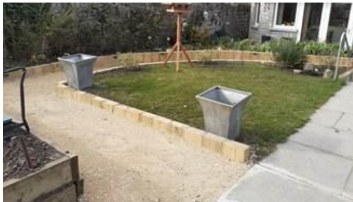
An accessible ramp installed to a resident's garden
